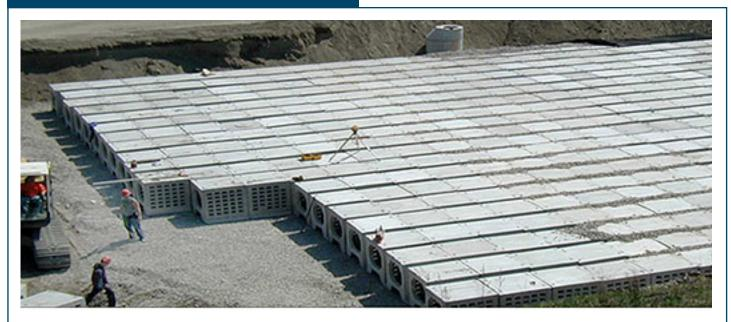
Any grouting that will inhibit the design/flexibility of the connector should be avoided.
